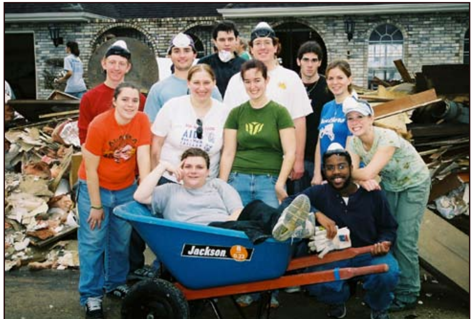
Service work was the centerpiece of Celebrate. A crew of Disciples and UCC students helped gut a northeast New Orleans home that had been flooded with eight feet of water. Getting grungy were, in the front row, Katie Griffin and Derrada Rashad Rubell-Asbell. Middle row: Lauren Short, Sarah Lornbach, Meredith Jackson, Dani McRaney, and Suzanne Castle-Rolen of University Christian Church in Fort Worth. Back row, from left, Jeremy Arnold, Clay Sauncy, Douglas Graham, Andy Castle, and Tony McMahon.
